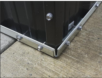
Corner Anchor Exterior - Bottom
